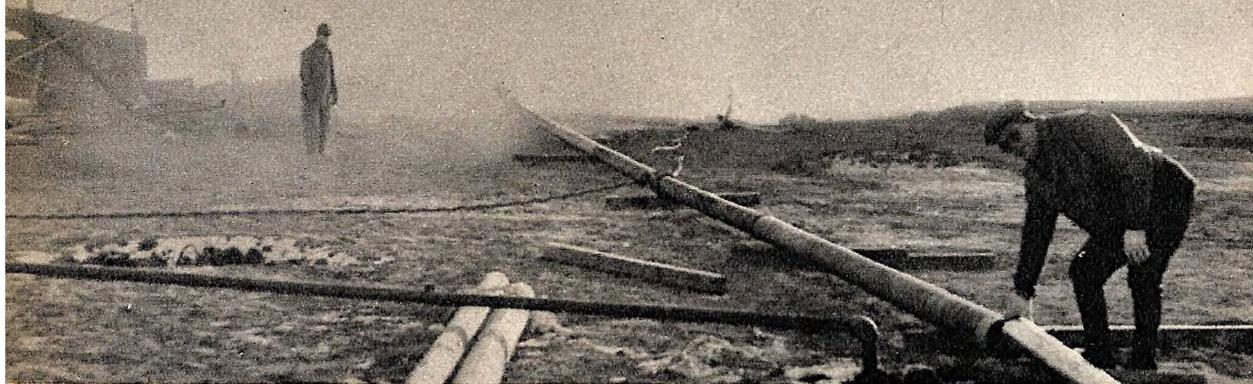
Lesh is shown placing nitroglycerin tubes in his pipe cannon. The torpedoes were drawn through the water cooled pipe and detonated at the mouth of the well.
