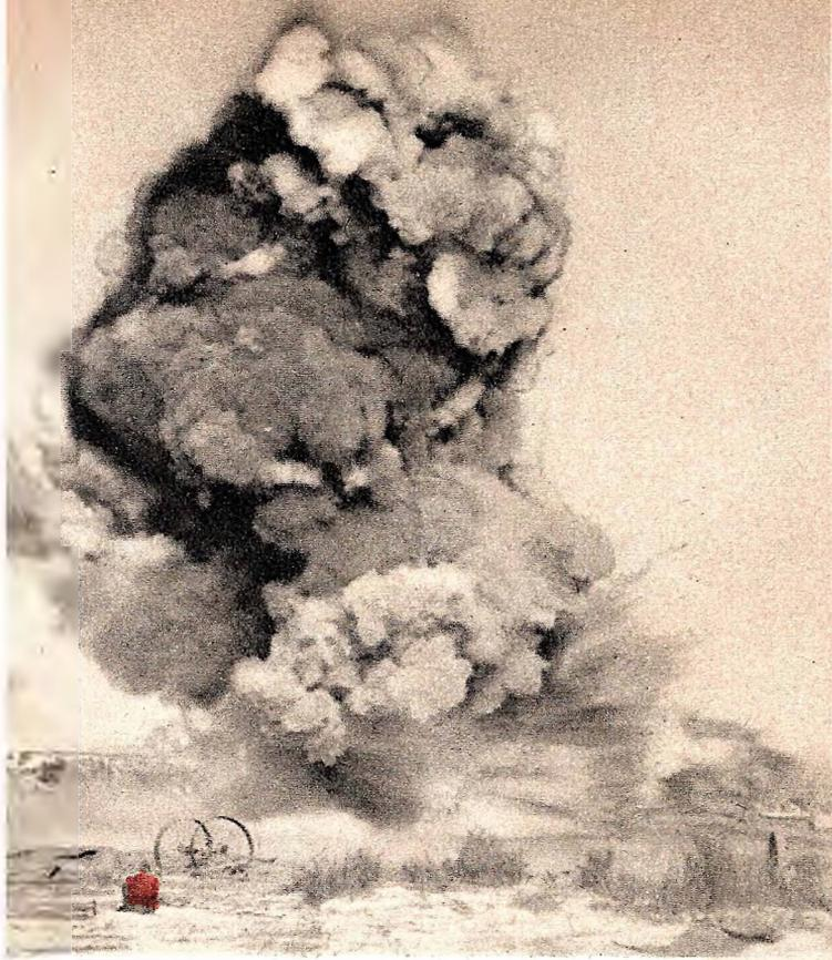
Twenty quarts of nitroglycerin were exploded to blow out the flaming well, pouring black clouds and tons of earth into the sky. Pipe cannon wheels are visible.
