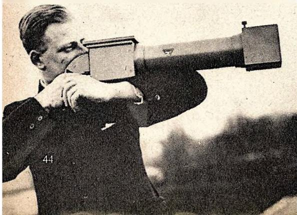
**D**EVELOPED as a safeguard against air attacks, which are usually unsuccessful unless the raiders can detect the lights of the city they are attacking, an "invisible" light lamp has been invented by Captain J. Bikker, a Dutch Army Intelligence officer. The lamp throws forward a light which can be seen only by a person standing directly in the beam. Neither the light beam nor the lamp itself can be seen, however, by anyone not in the line of the beam. No ray, not the slightest
