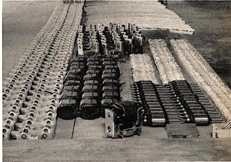
Above—Some of the parts used for the construction of the model subway system to be operated under the diorama buildings. Below—One hundred tiny street and traffic lights will add realism to the diorama. The traffic lights contain small red and green bulbs which will flash their colors in accordance with miniature traffic conditions.
