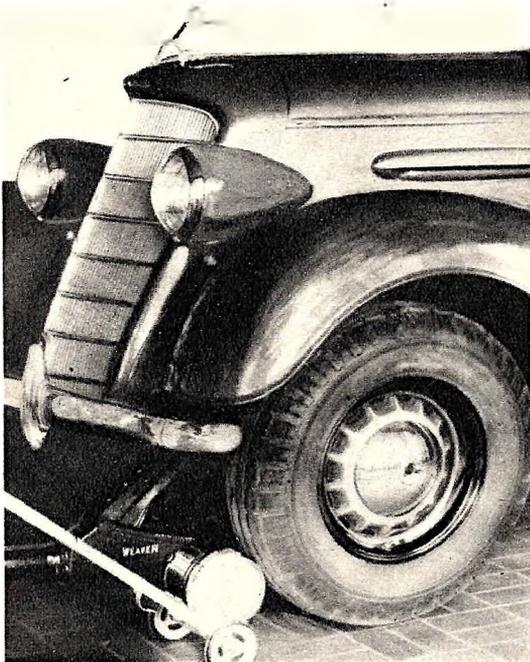
**T**HE testing machine shown under the car wheel eliminates the need for dangerous road tests or prolonged indoor testing when trying to locate an unbalanced wheel which causes a car to "shimmy" when speed is increased beyond a certain point.
