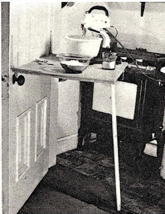
In position for use, the table is sturdy and will hold safely, most of the appliances used in the average kitchen. If a larger table size is desired, two legs may be necessary. Left — The drawing shows the dimensions of the top and leg.
