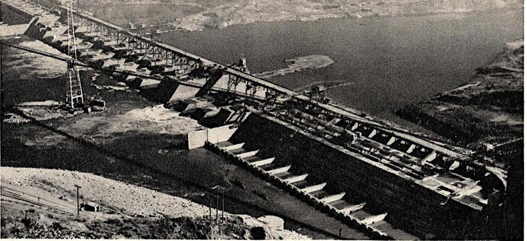
Grand Coulee Dam on the Columbia River in Washington (above) is about 50% completed. Cooling the tremendous heat liberated by the "curing" concrete is a major refrigeration problem. How it is being done is explained in the text below.
