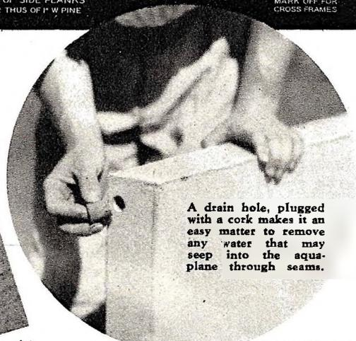
A drain hole, plugged with a cork makes it an easy matter to remove any water that may seep into the aquaplane through seams.
