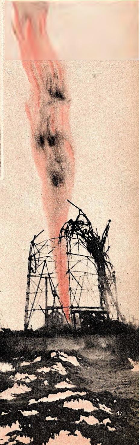
A glass blown rock striking the crown block caused the first fire that reduced the derrick to a twisted mass of steel. 60 million cubic feet of gas burned daily.
